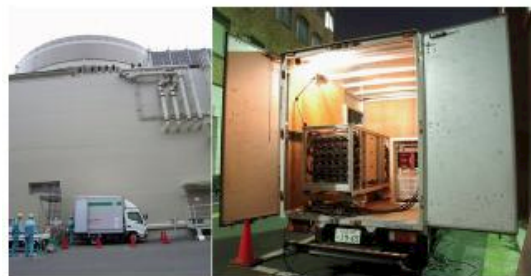
PANDA deployed in the van beside the reactor building of Ohi Power Station in Fukui, Japan.
