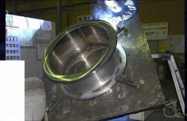
Welding on the connection port
